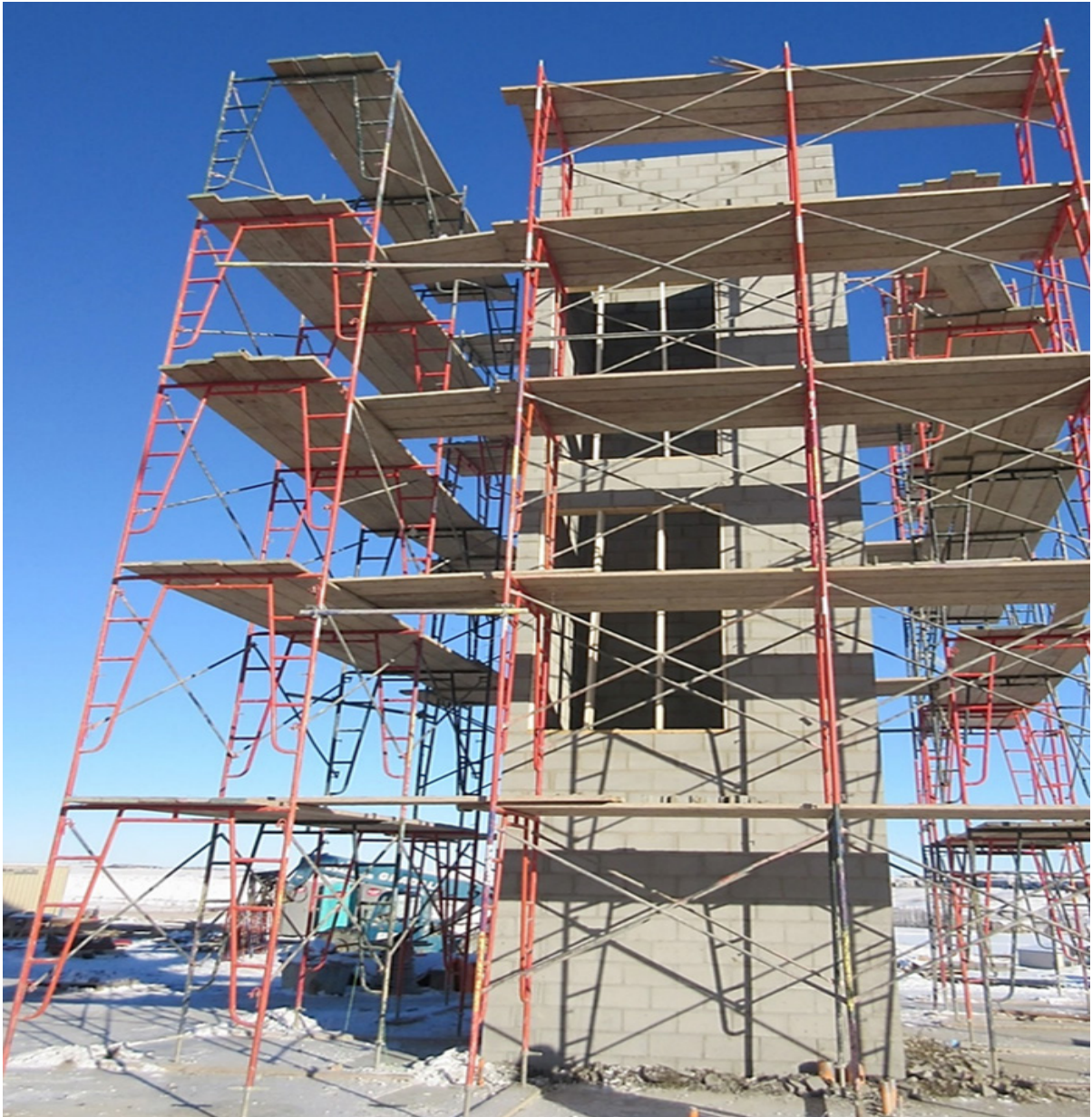
Figure 12: Elevator Shaft Permanently Detached from Wood Framing
