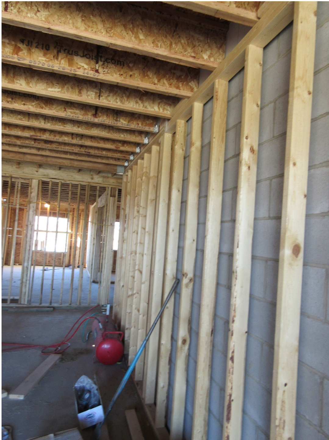
Figure 10: Elevator Shaft Permanently Detached from Wood Framing Under Construction - At Ground Floor
