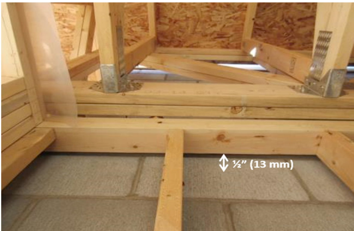
Figure 7: Elevator Shaft Permanently Detached from Wood Framing Under Construction - At Top Floor
