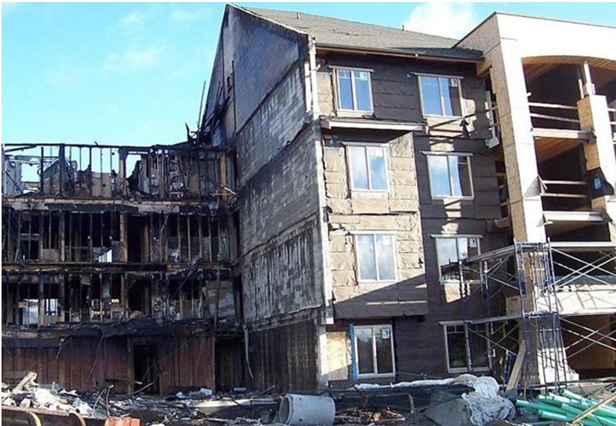
Figure 14: Block Fire Wall Laterally Supported After a Fire Event by the Wood-Framing
