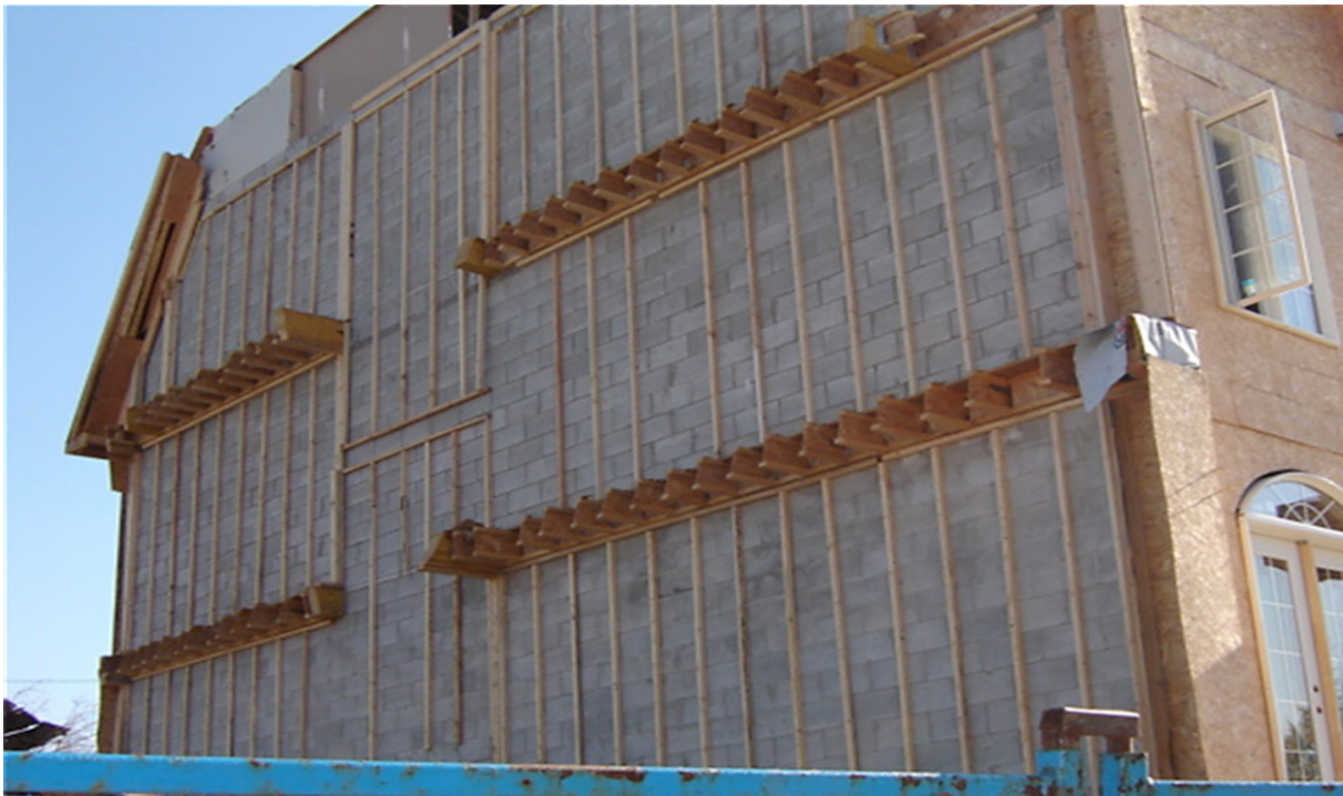
Figure 14: Block Fire Wall Laterally Supported After a Fire Event by the Wood-Framing
