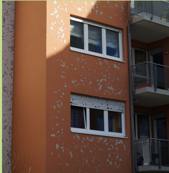
Hail can seriously damage low-durability wall cladding materials such as stucco and vinyl siding.
