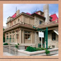
aimed at stopping and repairing deterioration to exterior masonry. The historic restoration concentrated on the building exterior. Un-doing changes made over the years and restoring the elevations to their original condition, especially the east elevation. The east or front elevation was finished with an articulated parapet and three cartouche panels.
